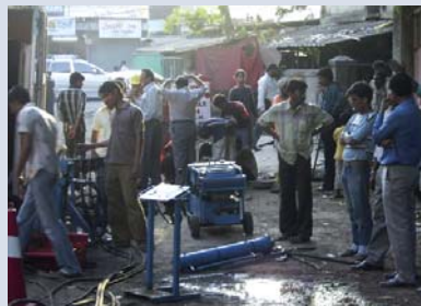
Preparing to work in a busy Mumbai street
