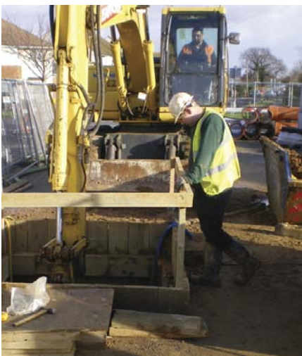
One of the three launch shafts dug for the project
