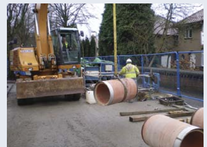
Preparing Naylor Denlock Clayware for installation
