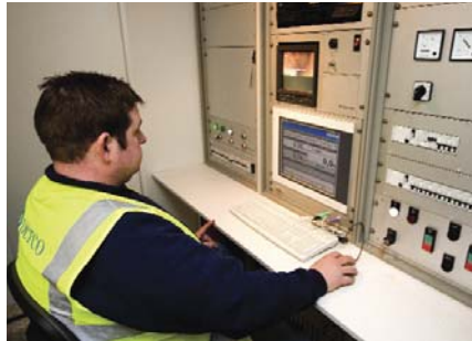
Lee at the controls of the EcoCIPP lining truck
