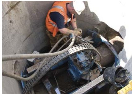
Auger boring operations from a 2.4 metre caisson shaft
