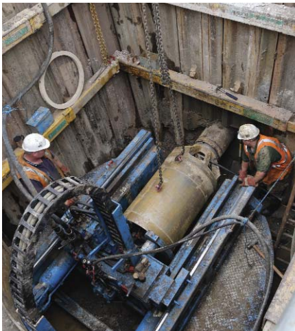
600mm extension arm is lowered into place in Perco's Bohrtec BM500 guided auger boring rig
