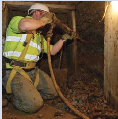
Dai Beer constructing a heading in Enfield, London
