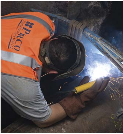
Welding lost steel casing during augering operations
