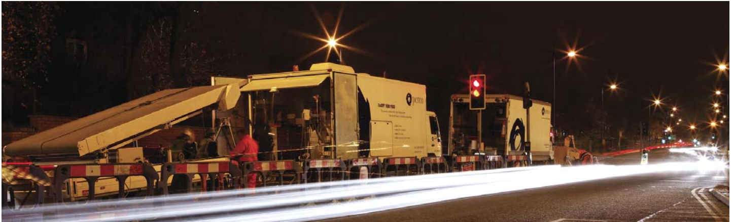
Our EcoCIPP lining team reline a Victorian U shaped sewer during overnight operations in Salford, Greater Manchester
