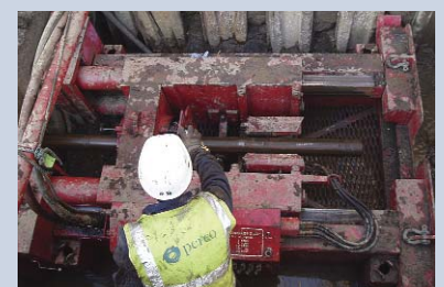
225 tonne rod puller set up for bursting
