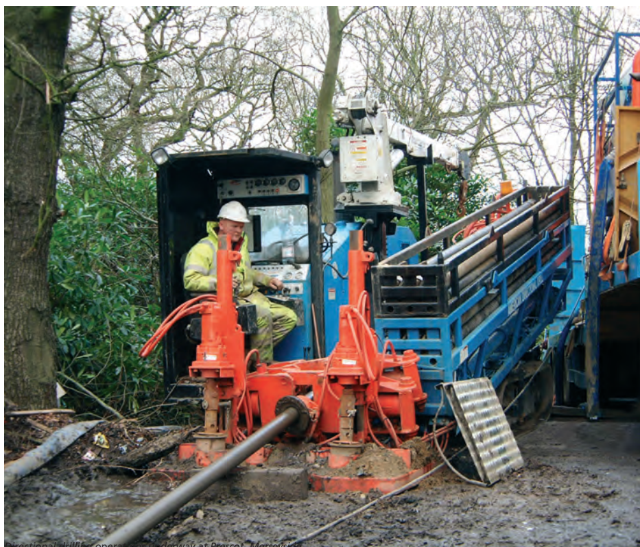
Directional drilling operations underway at Prescott, Merseyside
