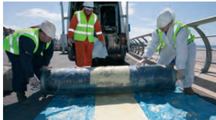
The patch liner is wrapped around an inflatable packer
