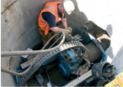
Guided auger boring works are carried out with a BM400 rig
