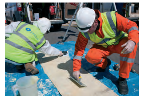
Resin is applied to a section of EPROS patch liner
