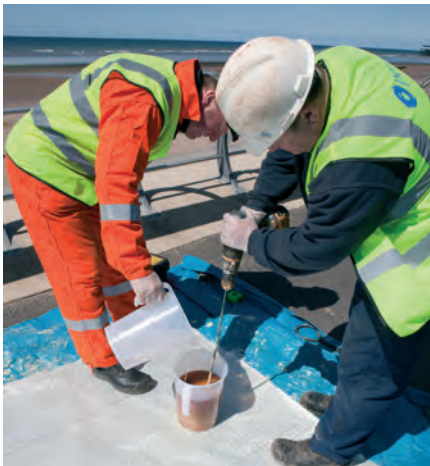
Preparing the epoxy resin for pouring on to the EPROS mat
