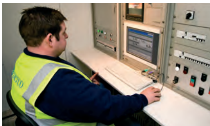
Monitoring progress of the EcoCIPP UV curing process
