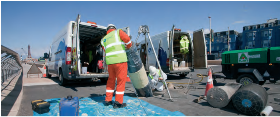
The patch liner and packer are lowered into the manhole
