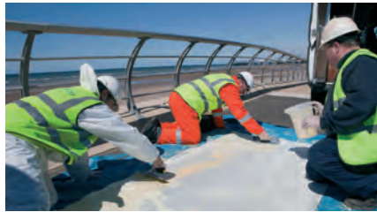
Resin is applied to a section of EPROS patch liner
