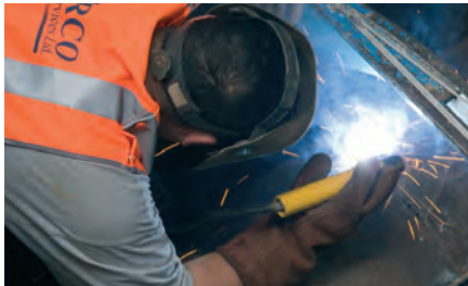
Welding sections of lost steel casing during augering
