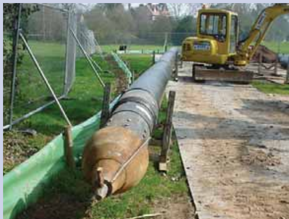
Pipe and towing head ready for installation
