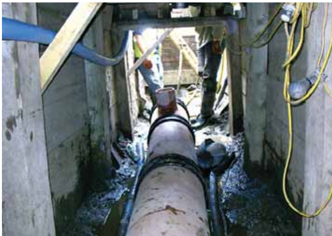
Clayware drains in position
