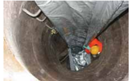
Installing an EcoCIPP liner
