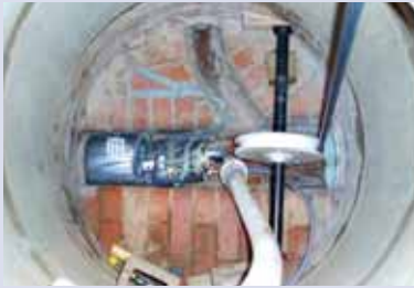
UV lining, Heathrow Airport
