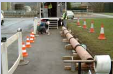
EcoCIPP demo day - lining trial in preparation
