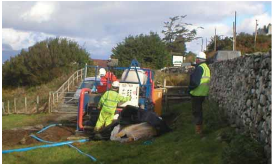
Cliff-top mud plant set up, Harlech
